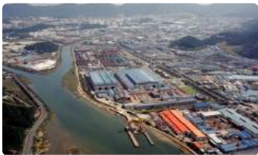
Completion of the Production-System Foundation
