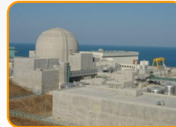
Emergency power generator
